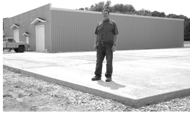
Ron Hanna, General Manager of classic Instruments, stands on the company's new permeable concrete parking lot which allows water to go straight through and not run off the surface of the parking lot. Underneath the concrete is 8 inches of stone to hold the water and let it dissipate into the ground, instead of sheeting off the top which creates erosion from the runoff. The 'green' lot is the first permeable concrete project of this size that is being completed this far north.
